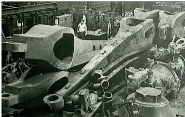
Figure 9. Gerberettes in the foundry Polig Heckel & Bleihart
