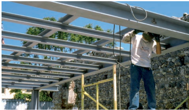
Figure 6. Structural steel solution with perception of construction system adopted for the coverage of the building.
