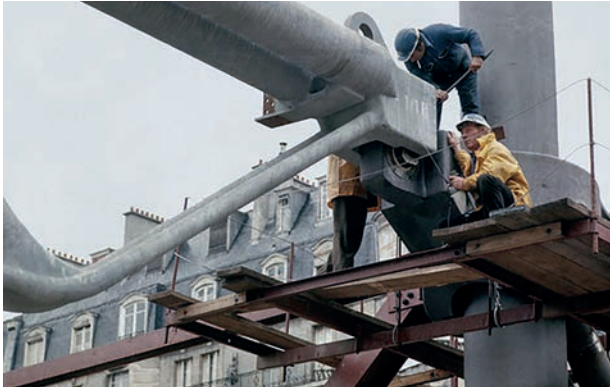
Figure 11. Operation of main beam attachment to the gerberette
