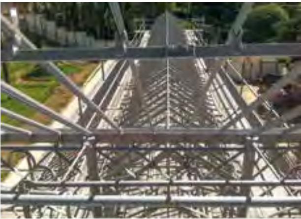
5. Photo during the process of recovery of the iron structure.
