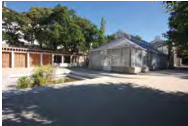
9. West side of the Tropical Greenhouse with lake in space coinciding with the old small greenhouse and Science space in situ on the left.
