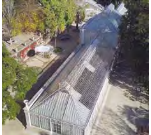
7. Aerial photograph of the Botanical Garden Greenhouse with small greenhouses on the upper platform to the north.
