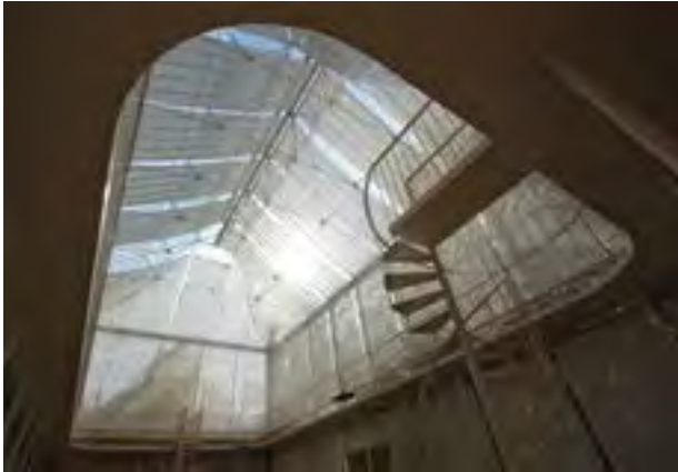
10. Photo of the main body of the greenhouse with active shading system.
