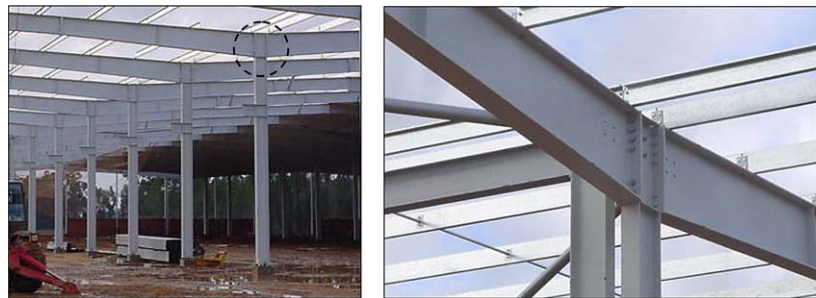
Fig. 1. Example of a pitched-roof portal frame joint.
